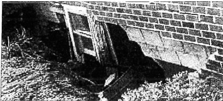
Rapidly rising floodwater can put extreme pressure on the foundation walls causing improperly vented structures to buckle and collapse. SMART VENTS® quickly and efficiently equalize the pressure and minimize damage.
